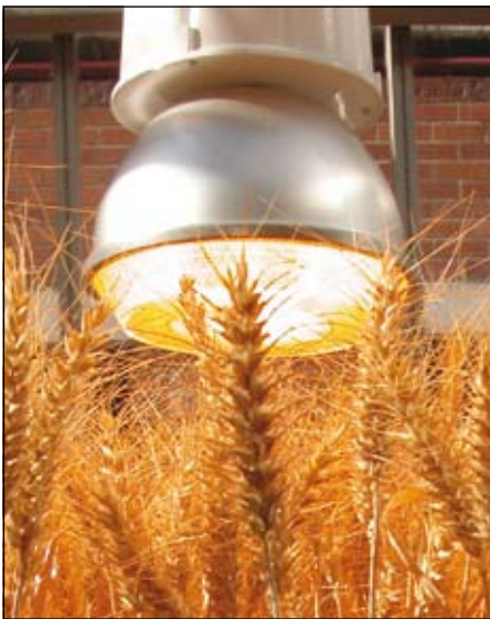
Continuous overhead hanging sodium lights give excellent canopy penetration. The greenhouse walls are fitted with light coloured panels to reflect additional diffused light back into the canopy.
